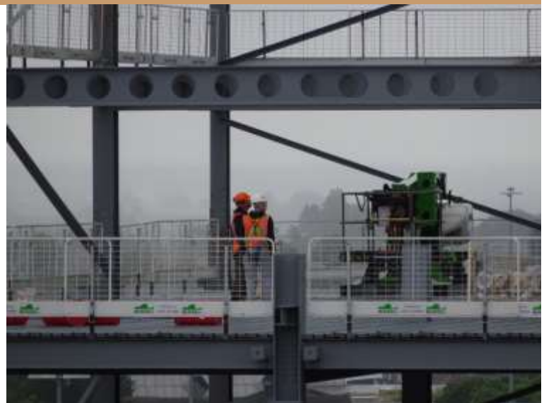
📍 Council offices at Friargate under construction
