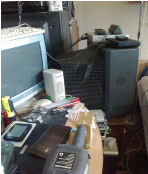
Hoard with electrical overloading
