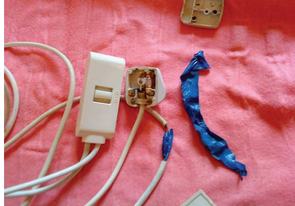
Faulty Electric Blanket
